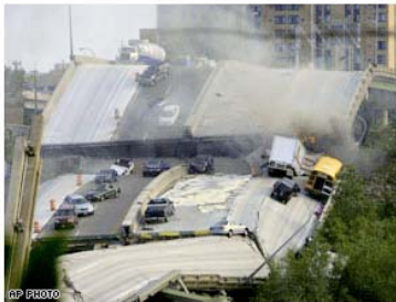
AP PHOTO Vehicles are scattered along the broken remains of the Interstate 35W bridge.
